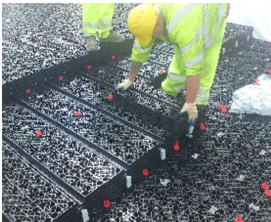
The new Enderby Park and Ride site (left). Workers are laying water storage crates. These crates form a chamber where rainwater that passes through the block paving and gravel layers is collected, so it can then flow into the nearby balancing ponds and gradually soak into the ground.
