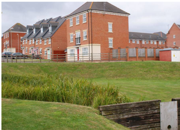
A modern development in Leicester which incorporates SuDS which runs throughout the site and discharges water to a nearby brook (left) and which also forms part of the Green Infrastructure of the development.
